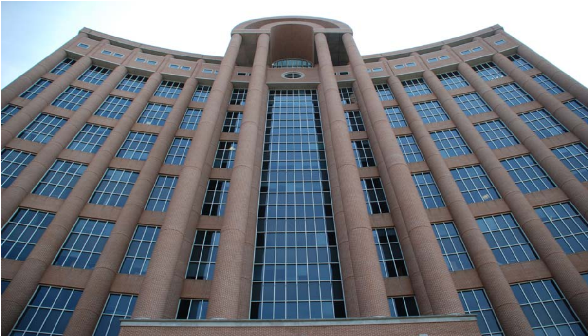
Tycon Towers By Philip Johnson
